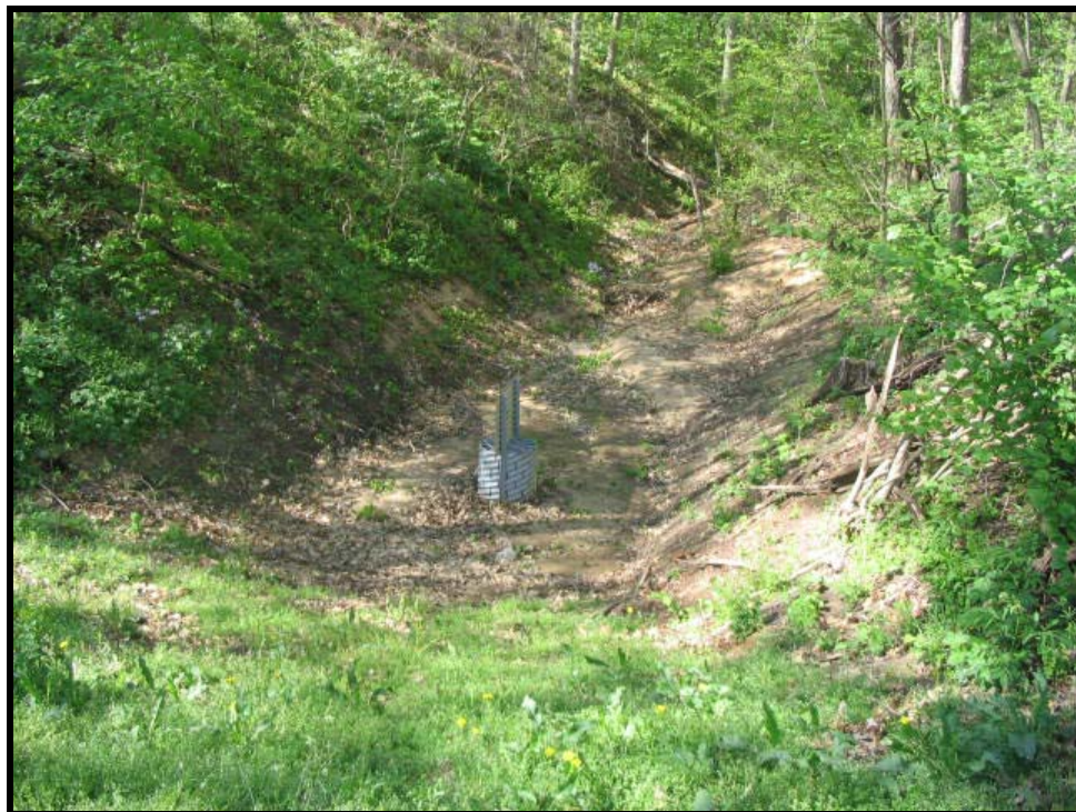
Figure 36. Sediment trap at the bottom of one of the ravines on the Limberlost Girl Scout Camp.
