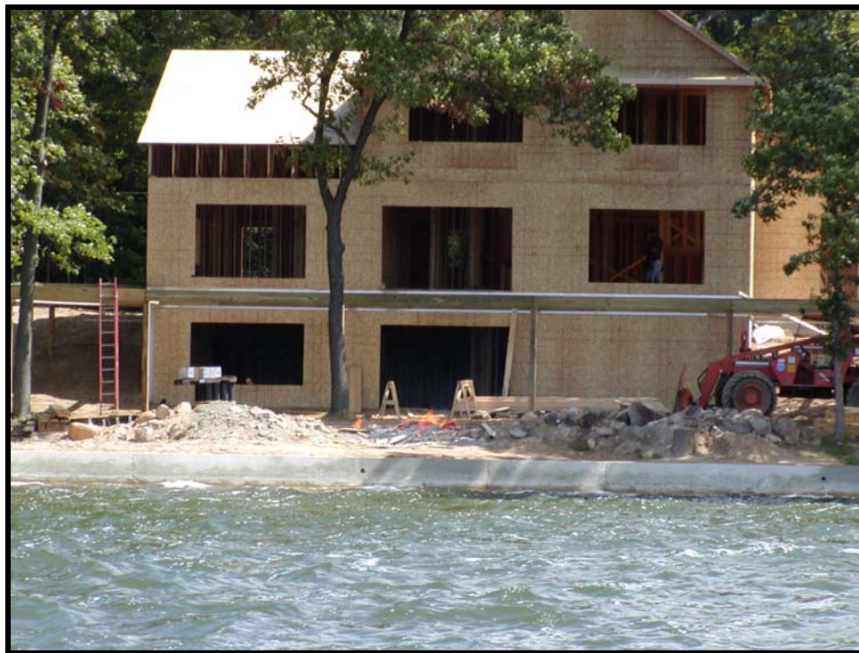
Figure 37. Development (or re-development) site along Dewart Lake that appears to lack silt fencing to protect the lake from on-site erosion. Additionally, construction debris is piled immediately adjacent to the lake and ash from the fire is undoubtedly reaching the lake adding to the lake's biological oxygen demand.
